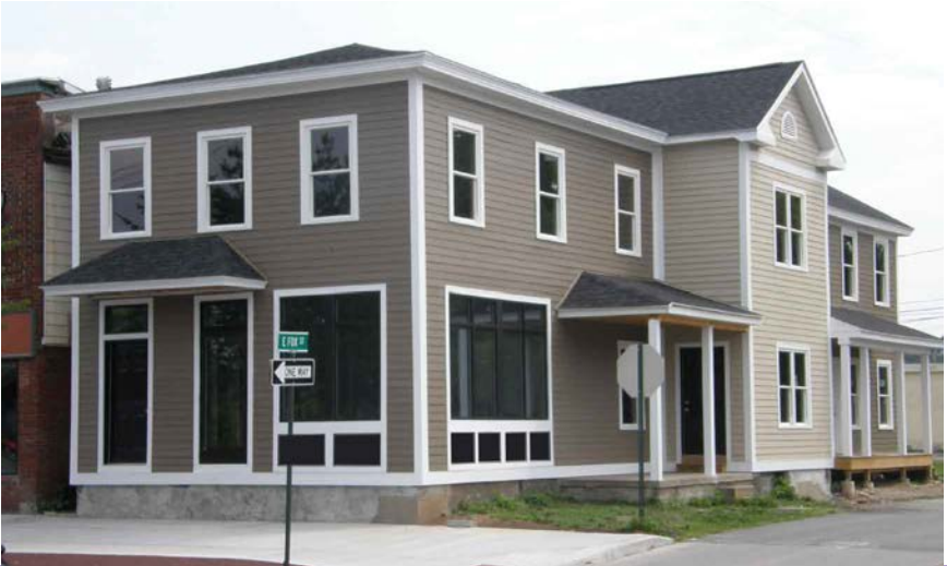
After Renovations Near Completion
