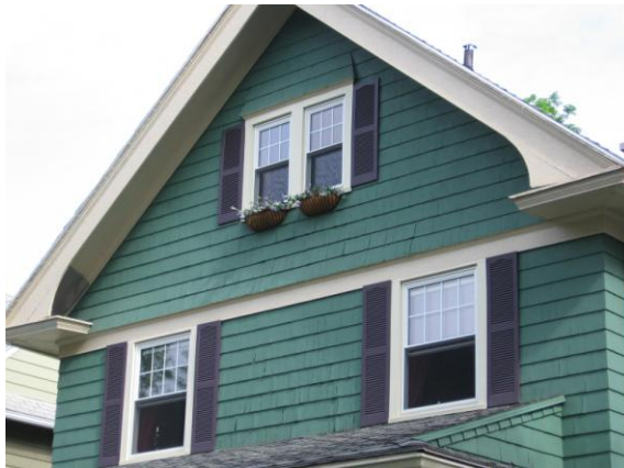
An example of replacement windows with interior grids and half screens.
