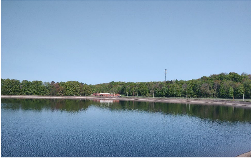
50 Million Gallon Filtered Water Reservoir
