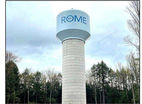
New 500k Gallon Elevated Storage Tank
