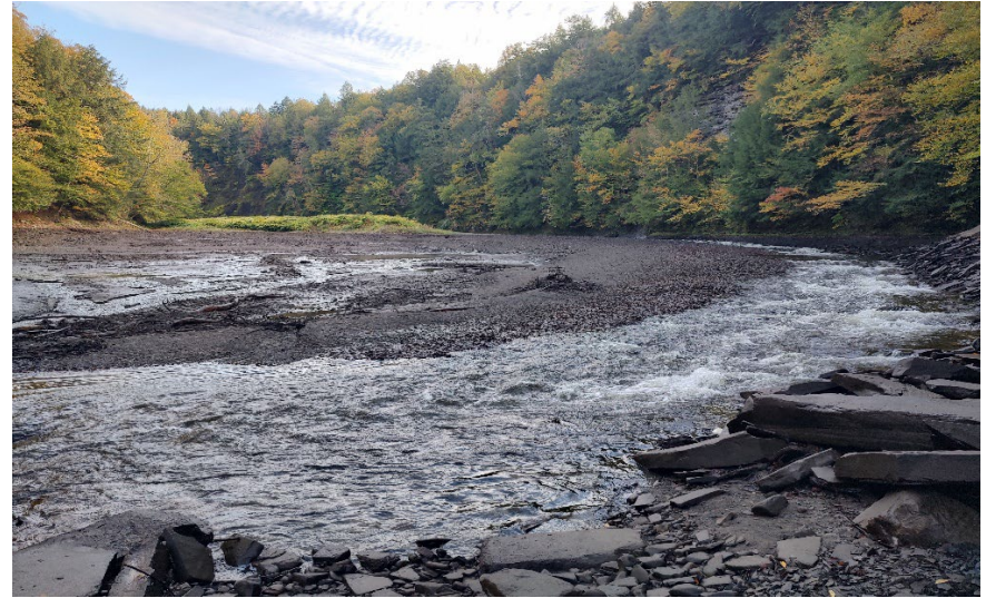
Kessinger Reservoir Drained for Maintenance
