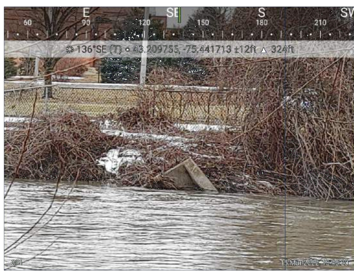
IMAGE OF EXISTING CULVERT OUTLET HEADWALL
