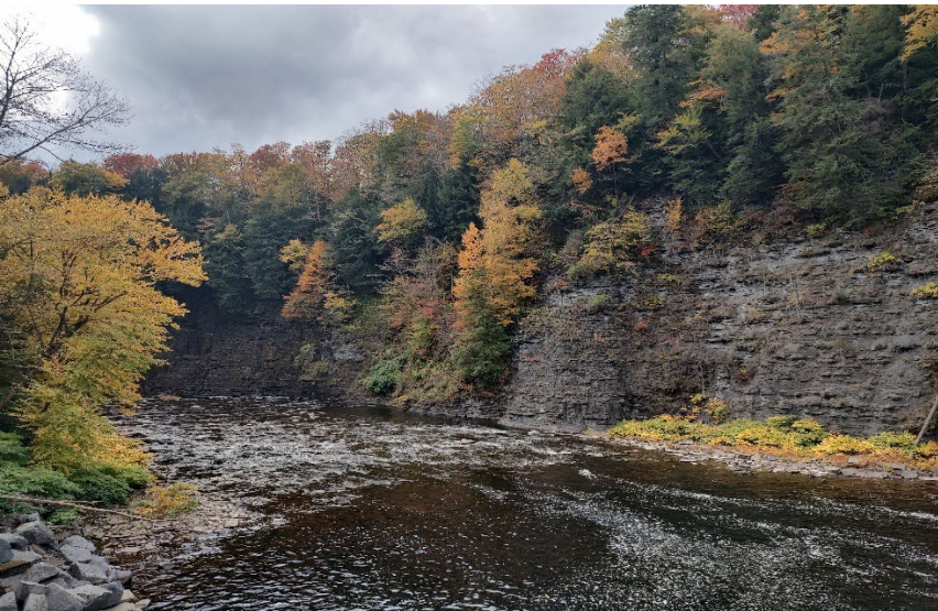
Downstream View at Kessinger Dam
