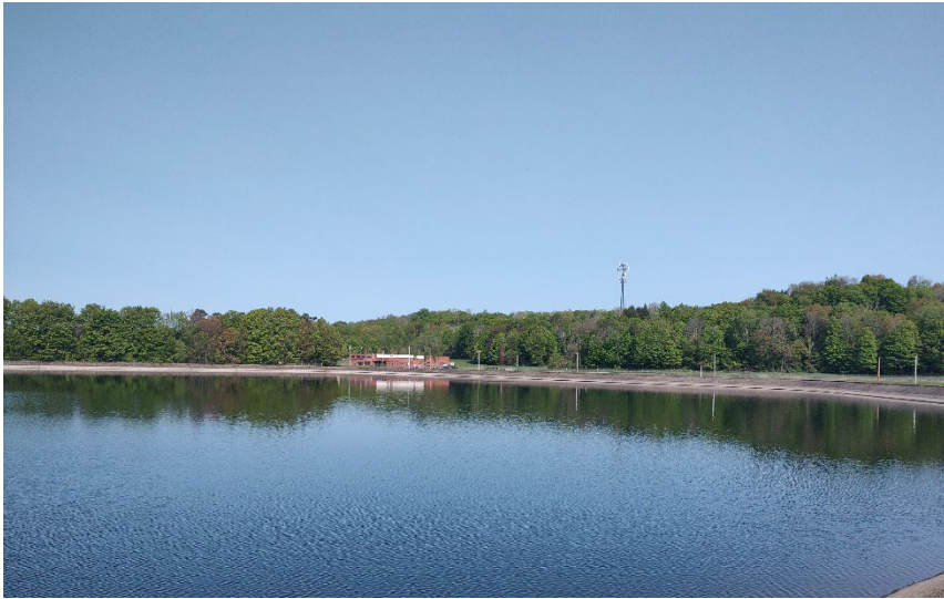
50 Million Gallon Filtered Water Reservoir
